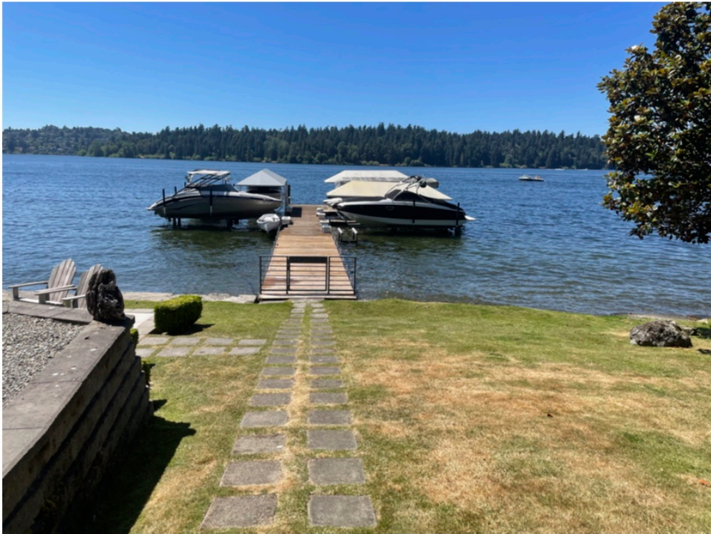
Photo 1 - Existing dock looking waterward.
